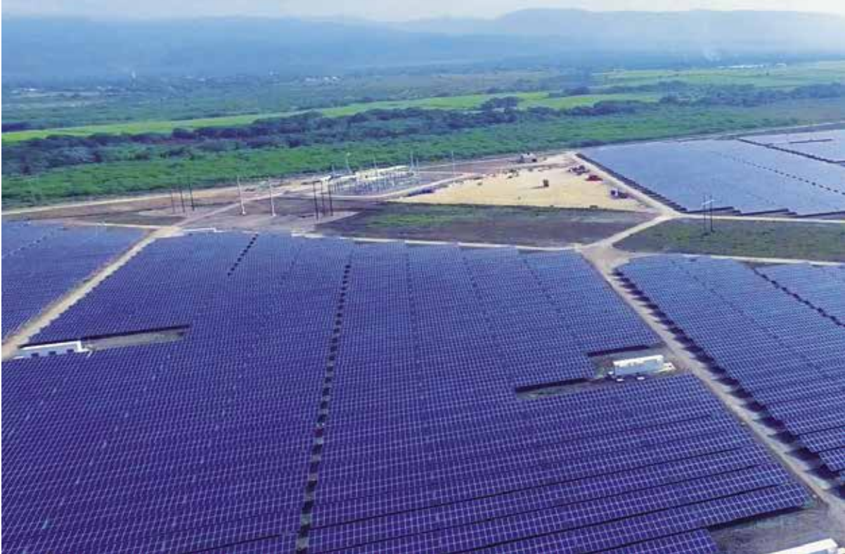
WRB Energy developed the 28 MWp Content Solar site in Clarendon, Jamaica.
