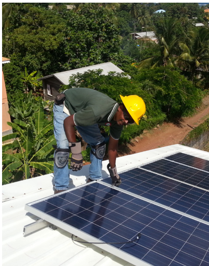
Grenlec solar photovoltaic (PV) rooftop installation in Grenada.
